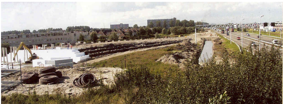
Figure 4 – Partly covered EPS-blocks belonging to EPS-1 approach road on the southern part of junction Sliedrecht-East
